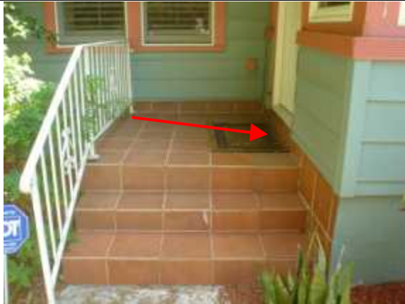
3. Monitor drainage at front stoop
